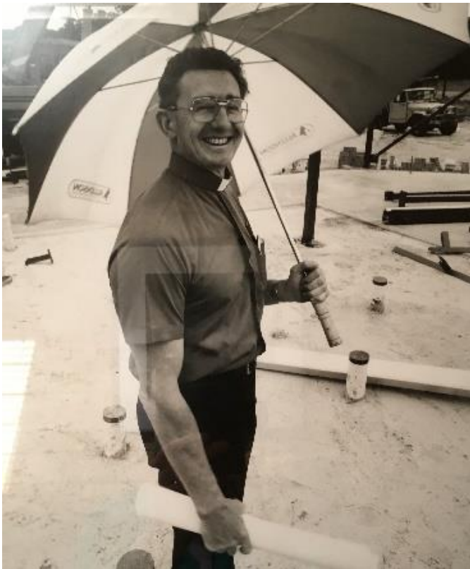
Building site at Menai parish
